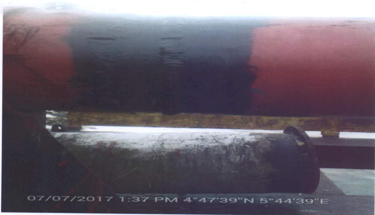
LEAK POINT REPAIRED
